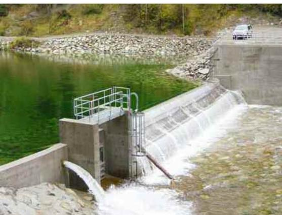
The low-elevation weir will be a definite barrier to migrating steelhead.
