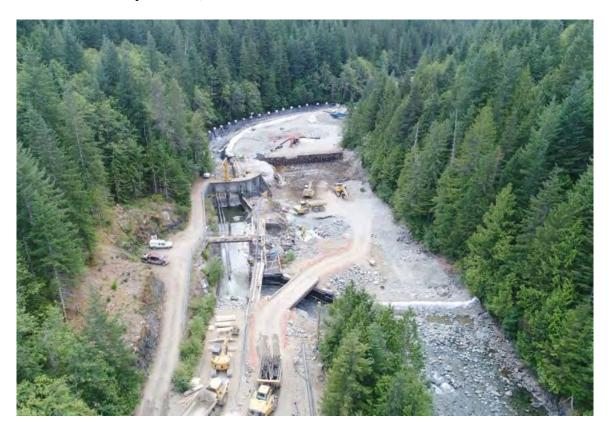
The course of the Salmon River was temporarily diverted to allow the removal of the timber crib diversion dam. Photograph by Emily Oliphant
